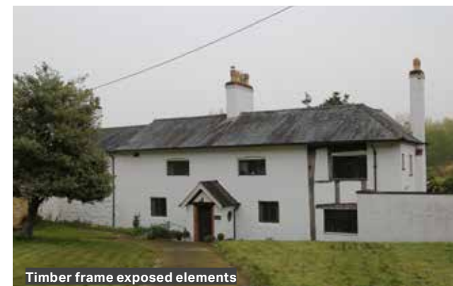
Timber frame exposed elements
