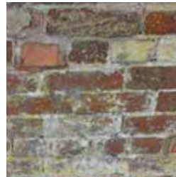
Lower section of wall
