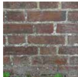
Former Manchester House wall
